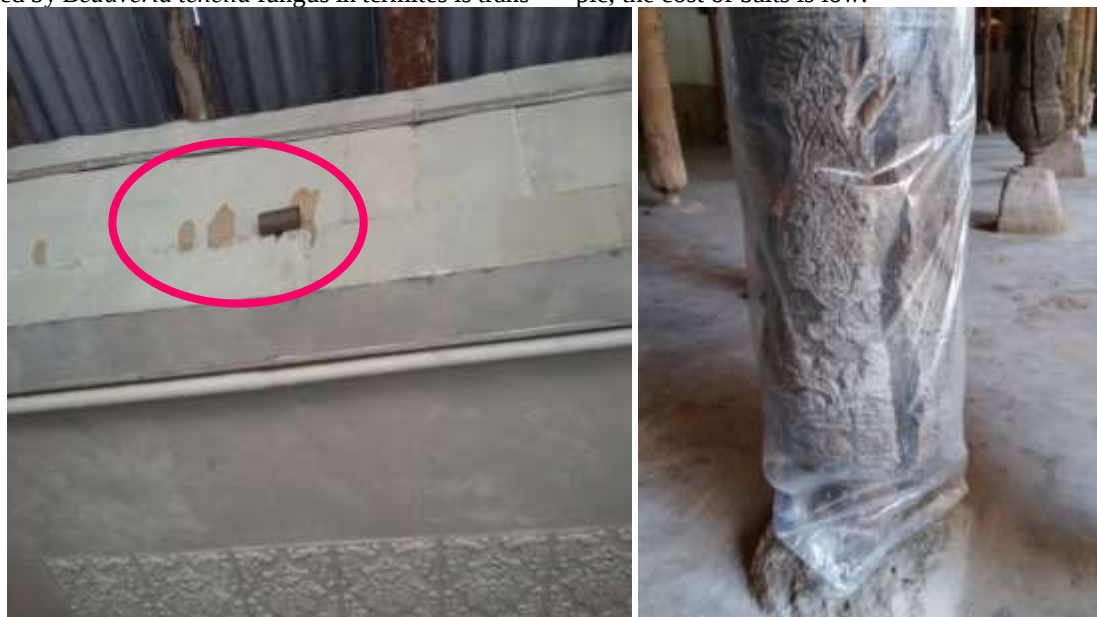
Picture 2 Installation of anti-termite baits
