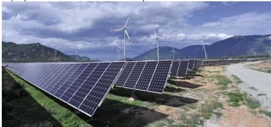
Figure 5. A general view of the hybrid SWPP.
