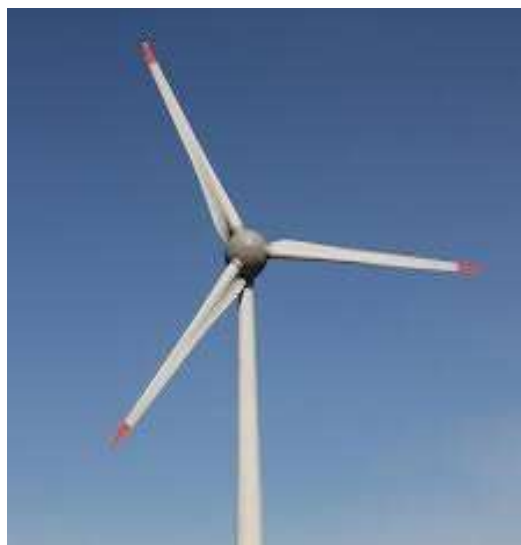
Figure 4. The general view of industrial three-bladed WPP.
