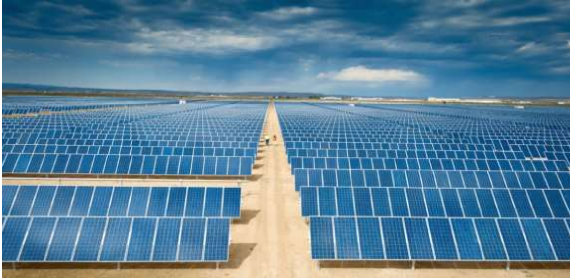
Figure 1. A general view of the solar power plant operating based on PVC.
