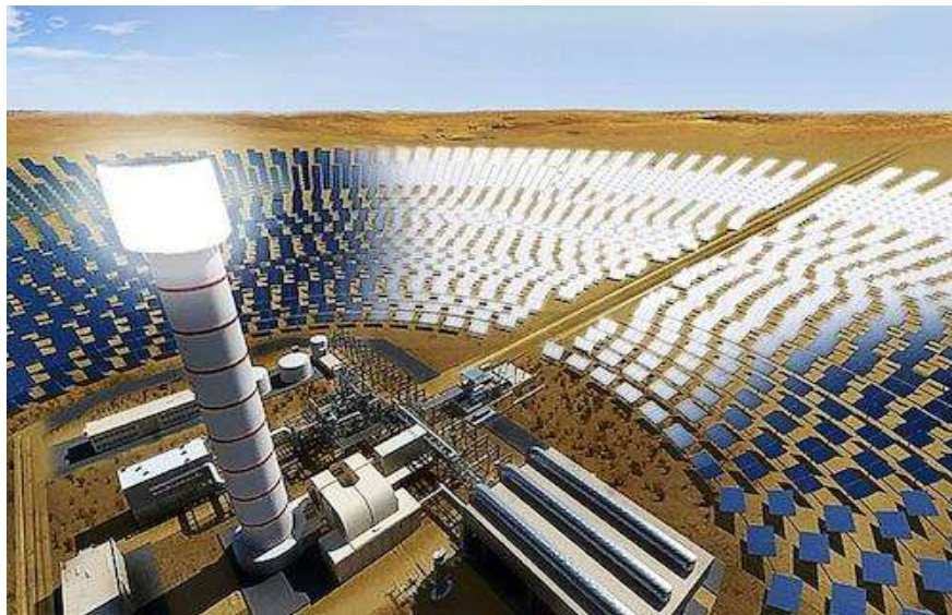
Figure 2. A general view of heliostat-based HTSPP.
