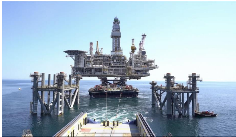
Figure 2: Delivery and installation of the top module of an offshore platform
