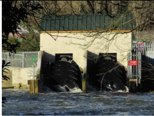
Figure 2. Micro-hydropower on the River Thames at Caversham Weir (Reading, UK) [21]
