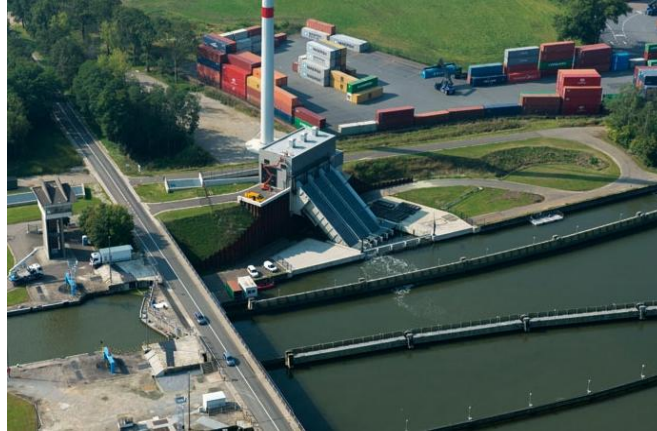
Figure 5. Combined hydropower-plant, pumping & turbine station on the Albertkanaal (Albert Canal) in Ham and Olen in Belgium [24]
