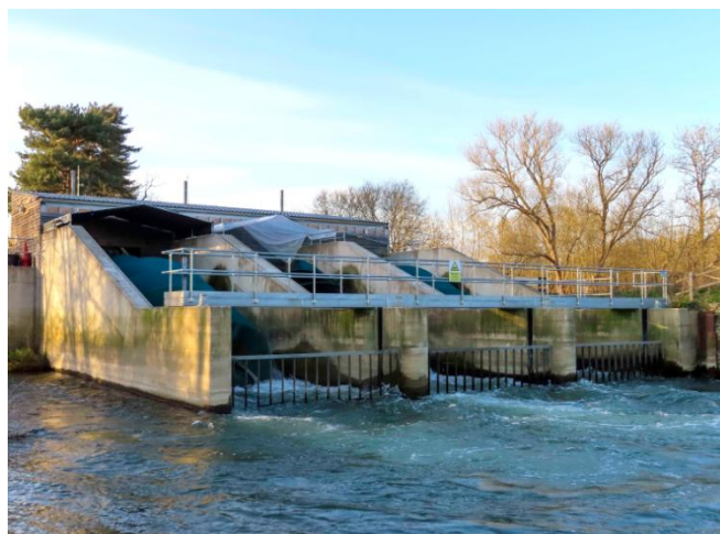
Figure 4. Sandford Hydro, the micro-hydropower plant located on the River Thames, in Oxfordshire, England [23]
